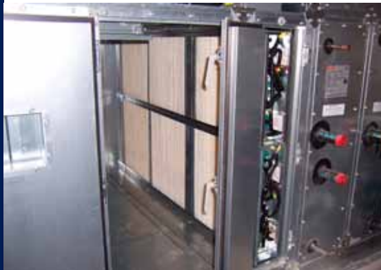
Laughlin AFB Fuel Systems Hanger Retro-Fit
