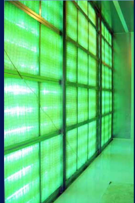
San Francisco Airport T2 Terminal Genesis Air Retro-Fit
